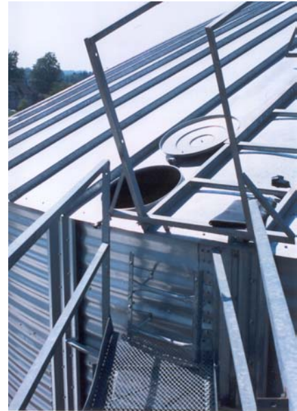
Figure 4. Open entry hatch at top of grain bin
